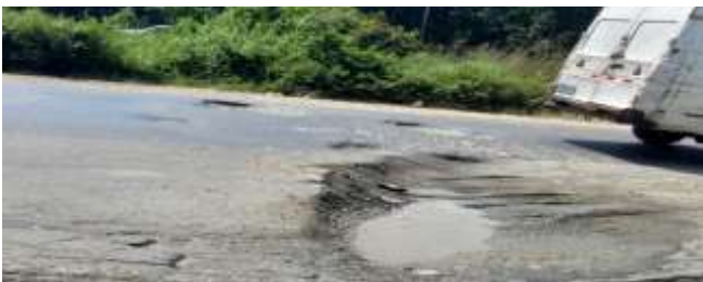
Plate 4: Failed Portion at Okolovu (Sand, Clay and Swamp)
