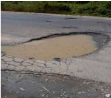
Plate 2: Failed Portion at Okuovwori (Sand, Clay and Swamp)
